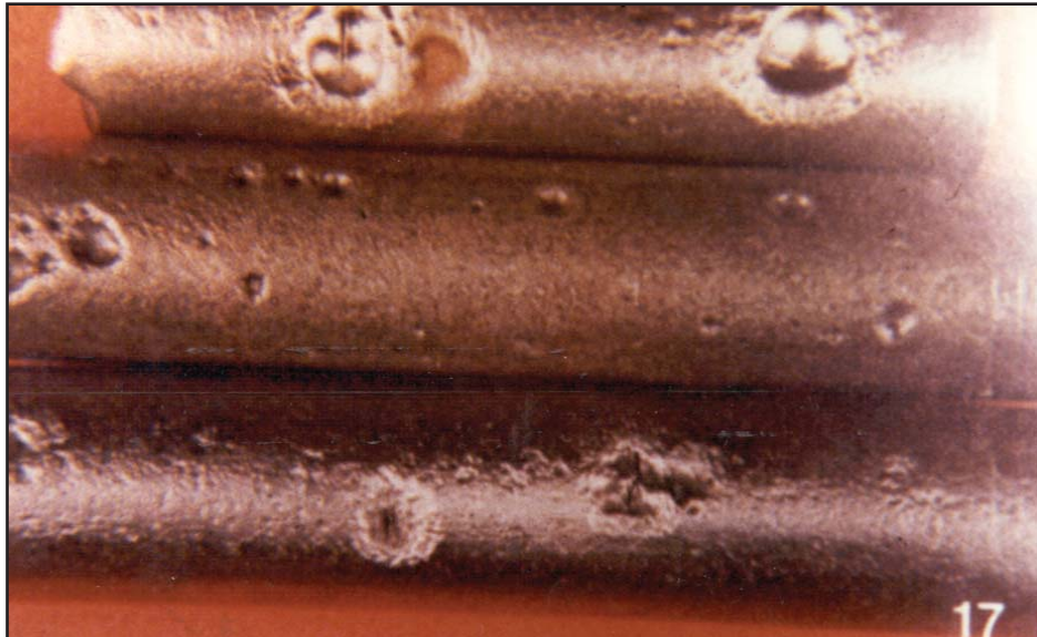
Figure III-1: Hydrogen Sulfide ( H_2S ) Corrosion
