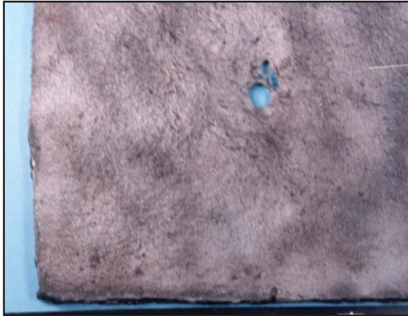
Figure VIII-6: Crude Storage Tank Failure Most Likely from Wet Oxygenated Soils
