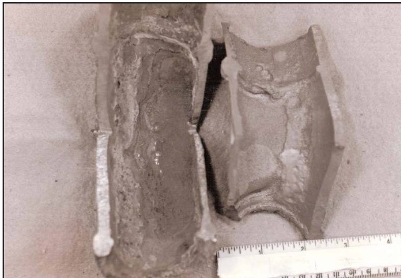
Figure I-38: Flow-Enhanced Corrosion in an Elbow
