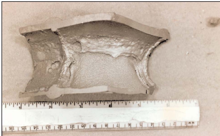
Figure I-39: Close-up Showing Severe Metal Loss
