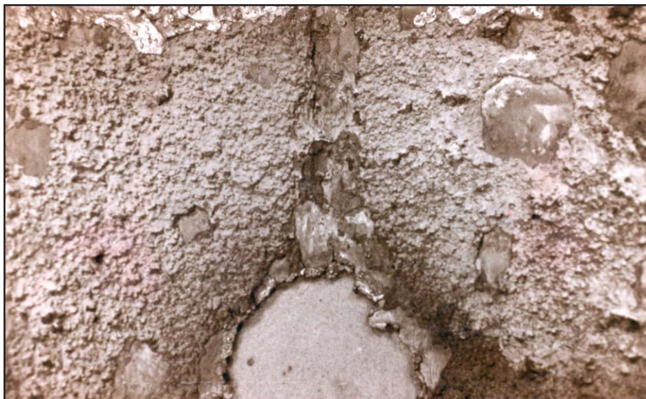
Figure II-7: Typical Rust-colored Deposits
