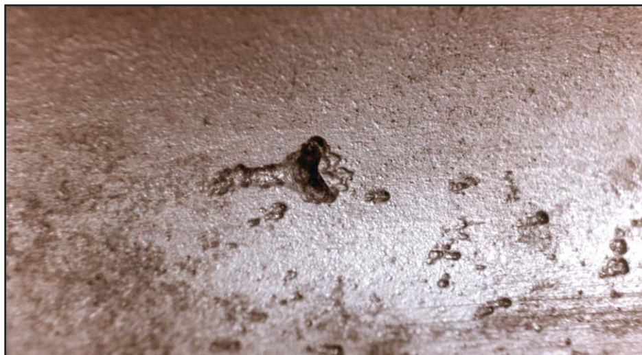
Figure I-33: Close-up View of Pit
