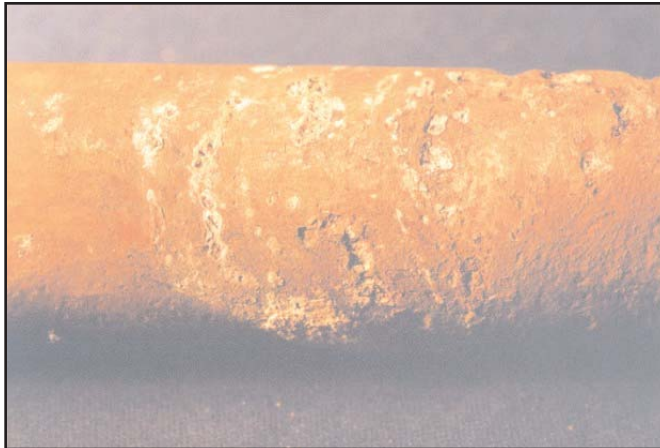
Figure IX-23: External Surface Depressions and Acidic, Light-colored Deposits
