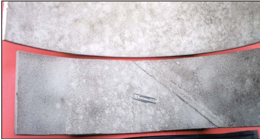
Figure VIII-8: Carbon Steel Product Pipeline Corrosion
