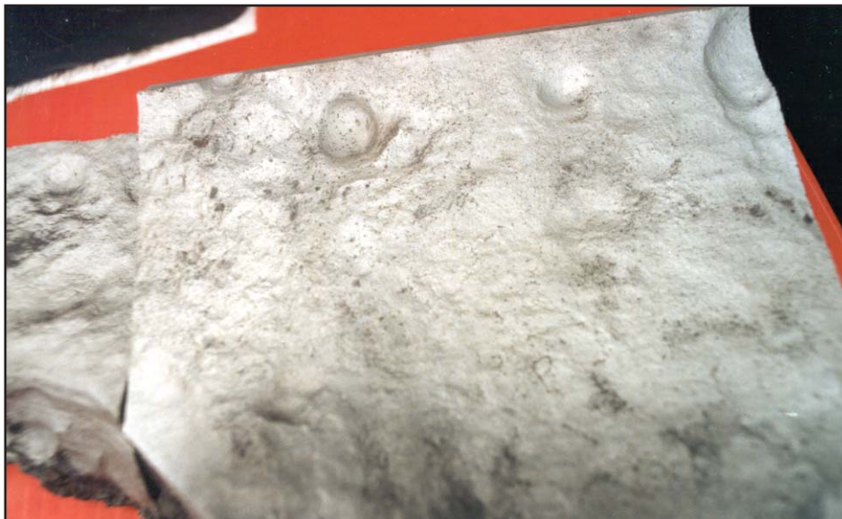
Figure V-2: Closer Inspection of the Pits
